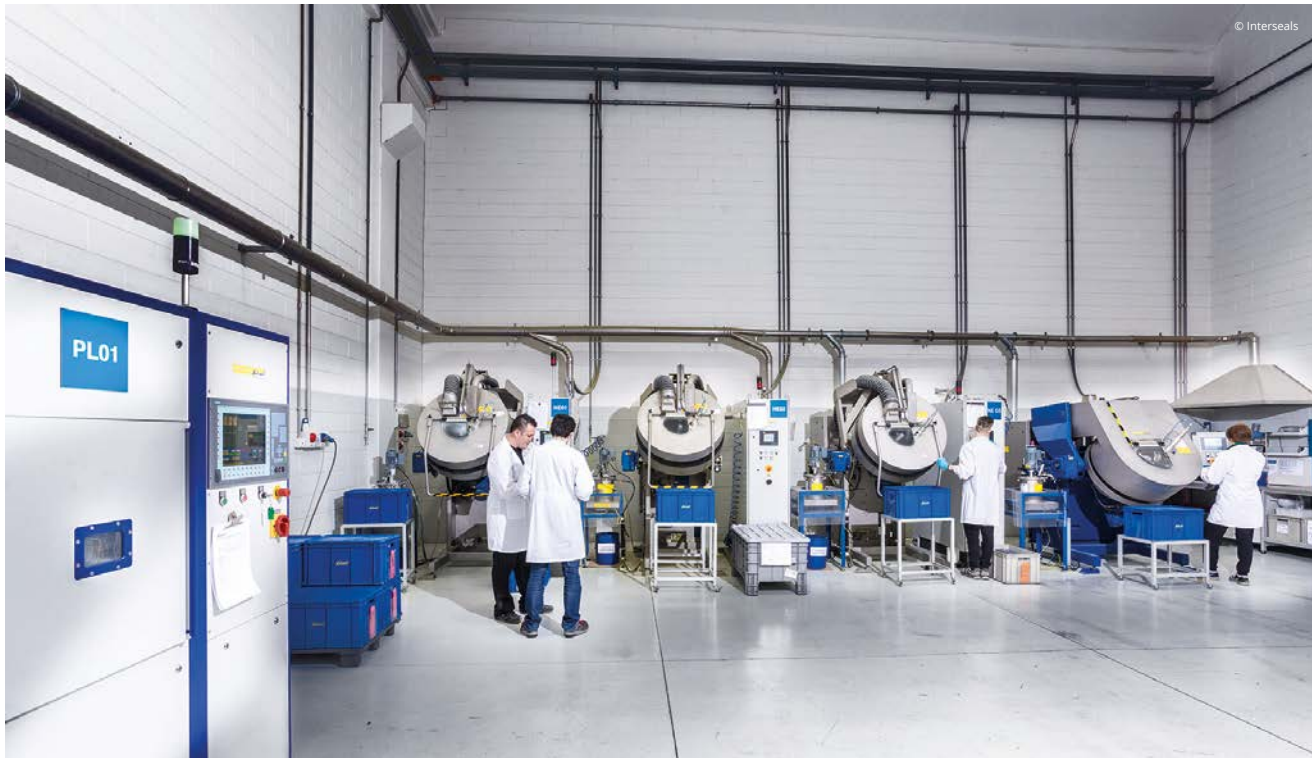
At its plant in Capriolo Interseals operates four Rotamat coaters. At Pol-Technology in Poland another three units are installed.
